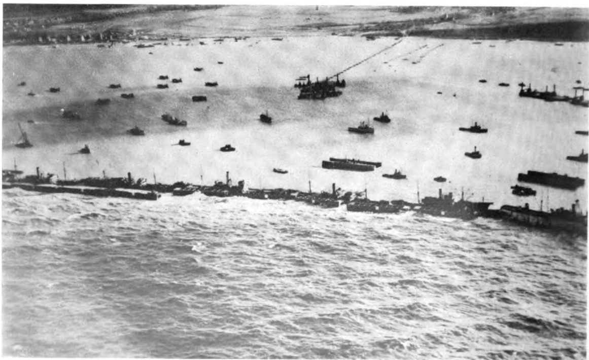
32. Mulberry harbour under construction. Note sheltered water
